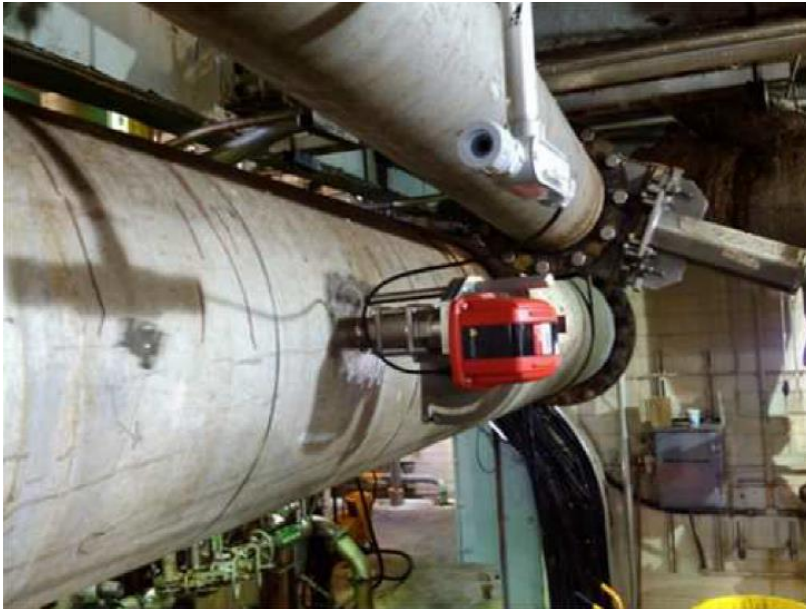
Figure 12: Bleach Load Transmitter In-Line
