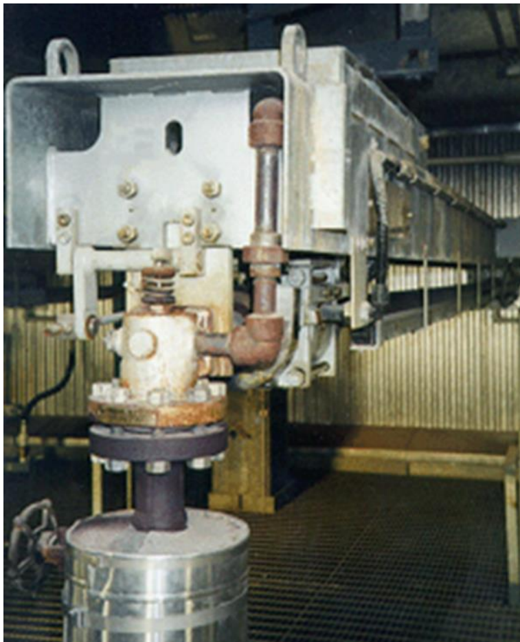
Figure 5 – Recovery Boiler Rotary Sootblower
